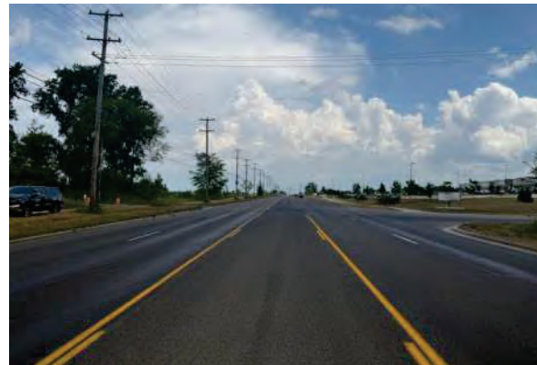
Eastbound 68th Street approaching Rapids Drive
